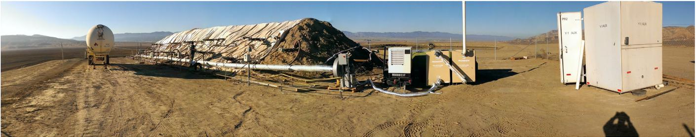
Ex Situ Thermal Desorption was used to successfully treat TPH-d and TPH-g from a former AST spill site in Central California. Affected soils were excavated and then placed “in a pile”, and Gas Thermal Remediation (GTR©) horizontal wells were placed into the pile during its three day construction. The piled soils represented mixed sands and high TOC soils, totaling a treatment volume of 77,692 ft<sup>3</sup>.
